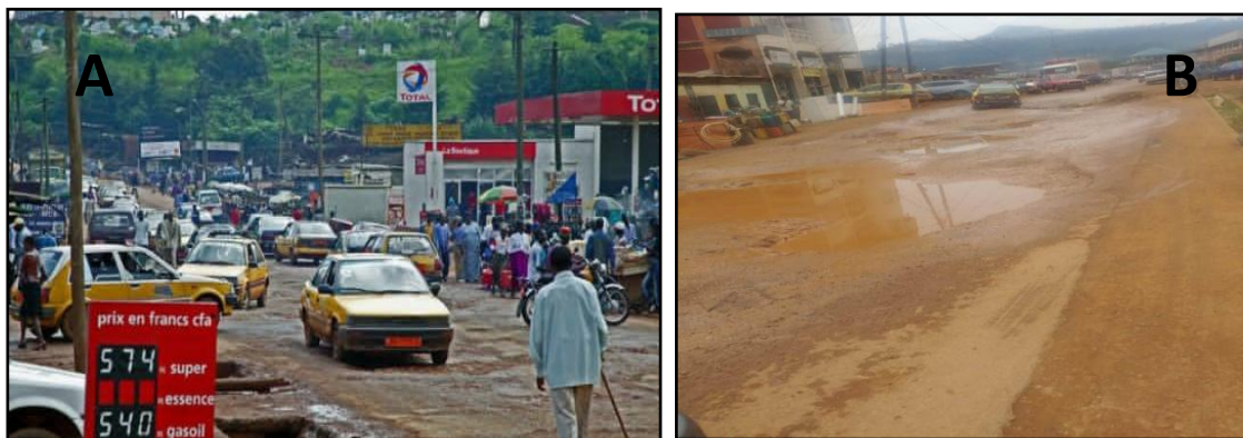
Plate 1: Damaged and pothole roads in the City of Bamenda
